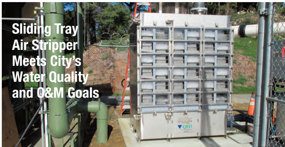
E-Z Tray air stripper occupies a small footprint behind large pre-treatment clarifiers.
